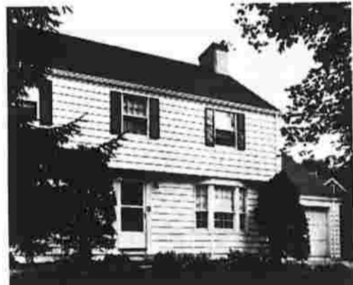
THE CHEERFUL LOOK OF VINYL SIDING — An occasional wiping with detergent and water keeps this GAF vinyl siding fresh and bright as the day it's installed.
